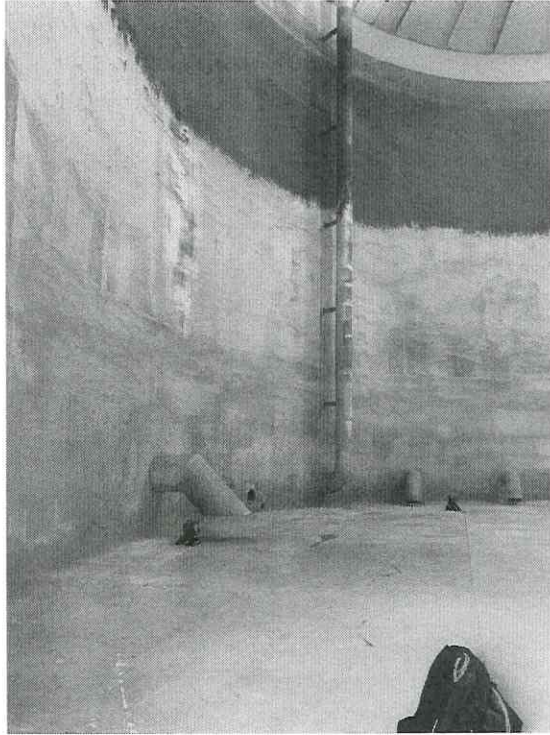
PHOTOGRAPH DESCRIPTION: View of Tank Wall
