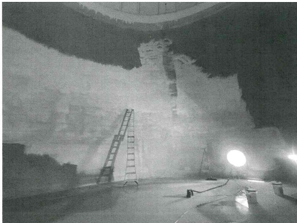
PHOTOGRAPH DESCRIPTION: View of Wall and Man-way Access.
